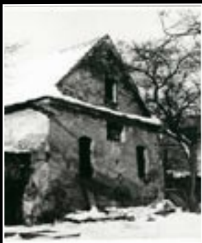
SYNAGOGUE EXTERIOR BEFORE DEMOLITION. 1980 PHOTO: JEWISH MUSEUM IN PRAGUE
